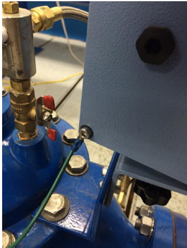
Figure 34: SPI Converter Grounding
